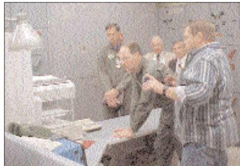
B. T. Knudsen explains the motor control center to Kehler. The center controls the power supply to the radar used at the 20th SPSS.
