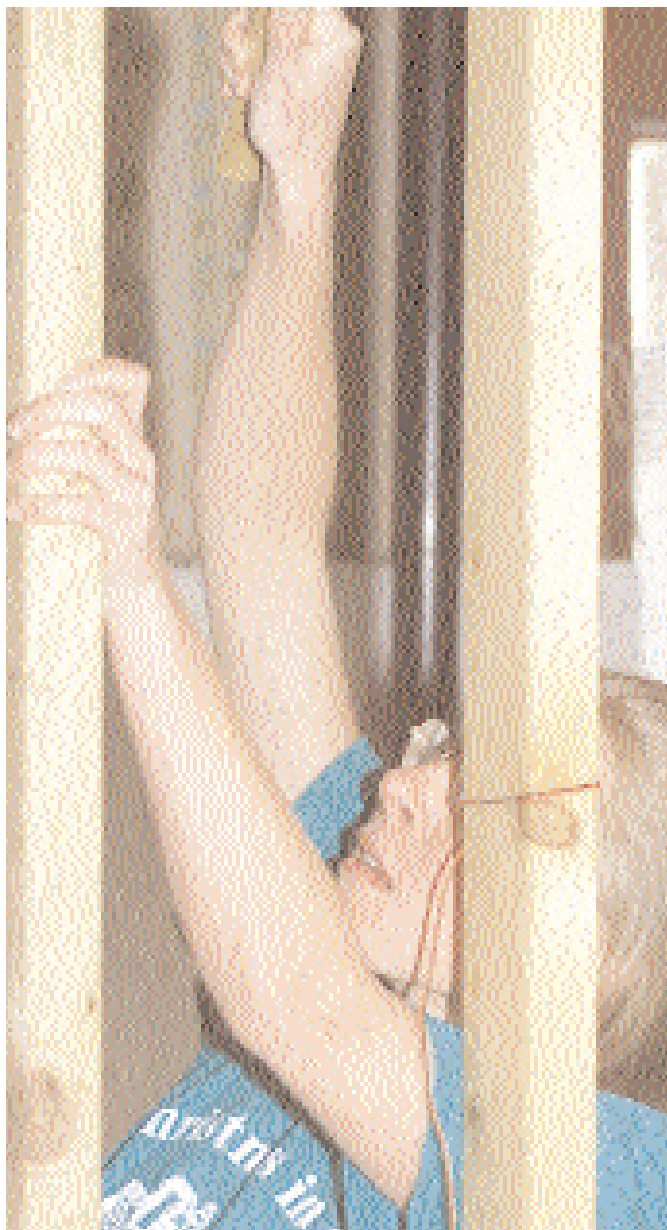
Remodeling and repair tasks accomplished by Peterson volunteers during the "Rebuilding Together with Christmas in April" project also included framing walls in preparation to hang new sheetrock, safety-proofing old trim, prepping new door trim, and hanging new doors.
