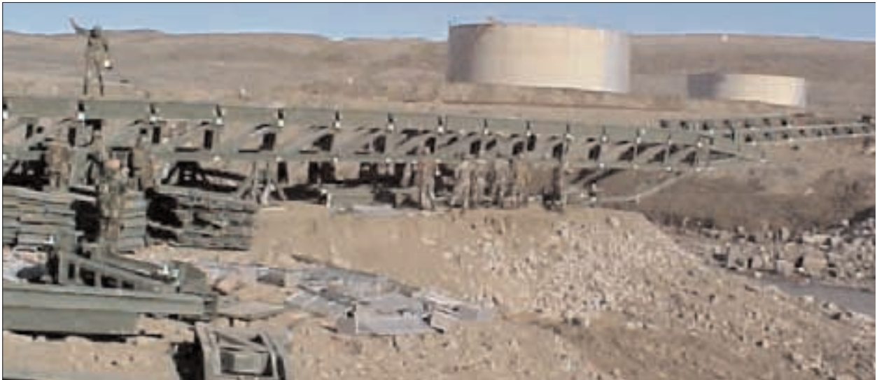
Above: Members of the 62nd Engineer Battalion from Fort Hood, Texas, put the finishing touches on the temporary bridge before moving it into place. The original bridge was destroyed by recent floods. Below: An Army supply truck drives over the bridge to a test it to make sure it is ready for traffic.
