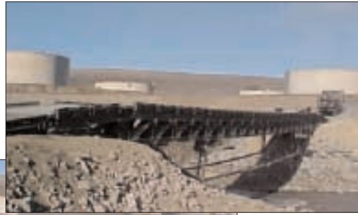
Left: The temporary bridge site before construction at Thule Air Base, Greenland. Above: A truck approaches the finished medium-girder bridge.
