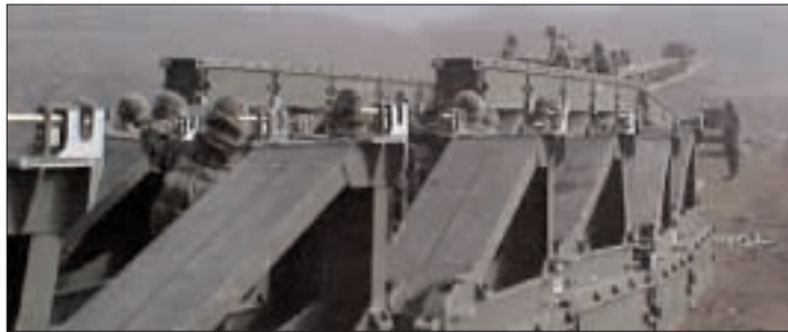
Above: Engineer Battalion members work on the temporary bridge as it extends into the fog. Left: A crane lifts one end of the bridge, moving it into place. Right: Soldiers assemble the medium girder bridge before extending it across to the opposite bank.
