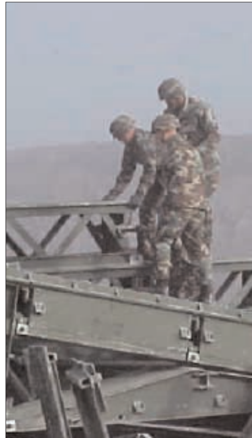
Above: Engineer Battalion members work on the temporary bridge as it extends into the fog. Left: A crane lifts one end of the bridge, moving it into place. Right: Soldiers assemble the medium girder bridge before extending it across to the opposite bank.
