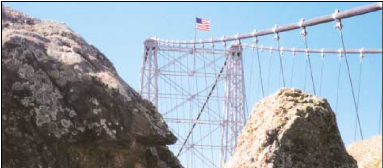
Cables used in the Royal Gorge Bridge construction are composed of 2,100 strands of galvanized wire. The towers are 150 feet high.
