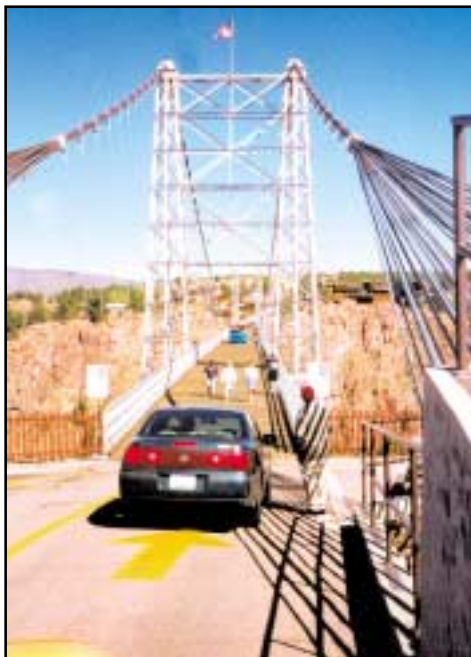
Visitors can cross the bridge by car, walking or riding the blue shuttle. More than 1,200 planks make up the floor of the Royal Gorge Bridge, which spans the gorge.
